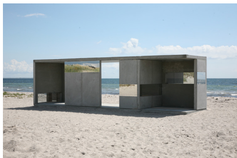
Gazebo , 2015 240 x 960 x 240 cm In situ cast concrete base, custom cast concrete elements, 2-way mirror glass, glass fittings, drainpipes, steel mountings. Art in Sunshine , ARKEN Museum of Modern Art
